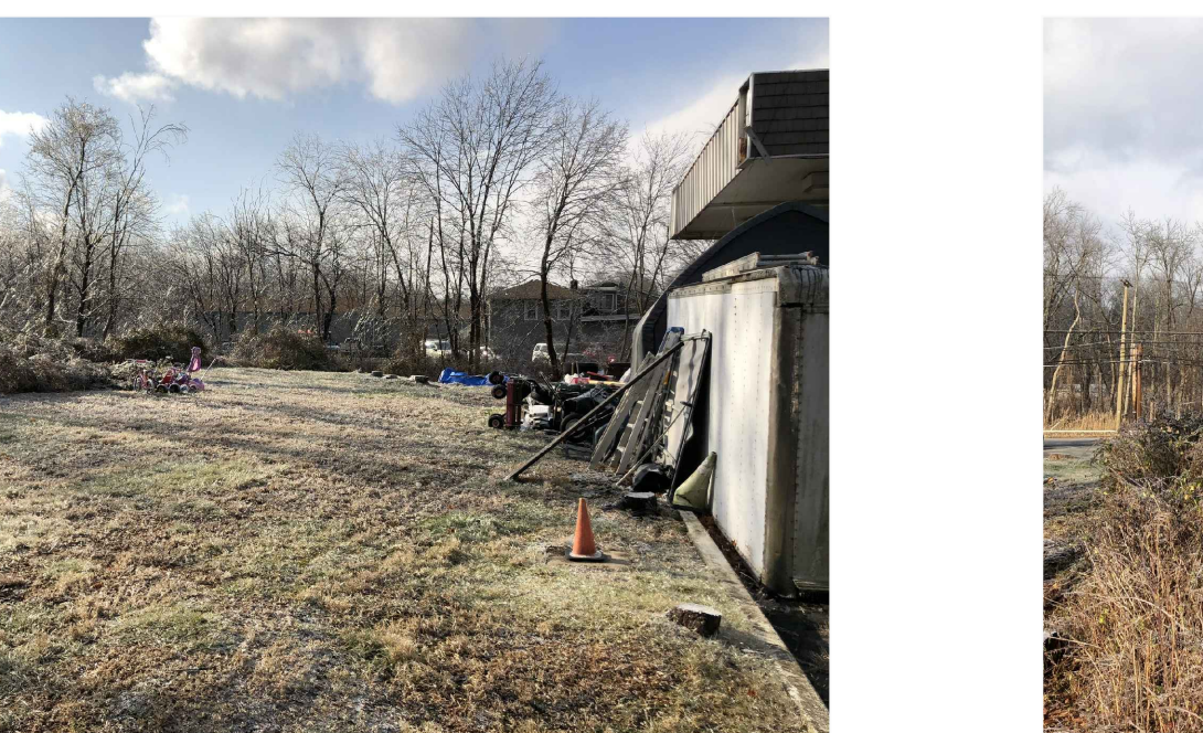
4 VIEW WEST TOWARD AREA OF PROPOSED ADDITION ADJACENT TO EXISTING STRUCTURE. AREA TO LEFT IS THE MITIGATION AREA.
